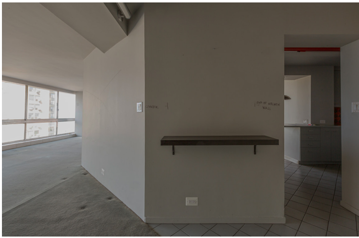
1 Kitchen Looking East
